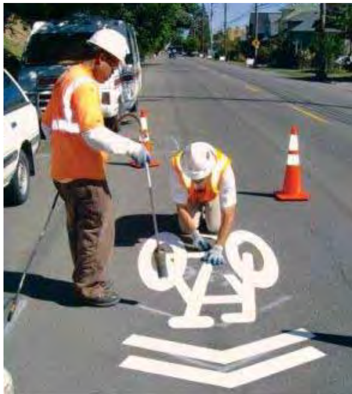
A shared lane can be installed by simply painting a "sharrow" on the street.
