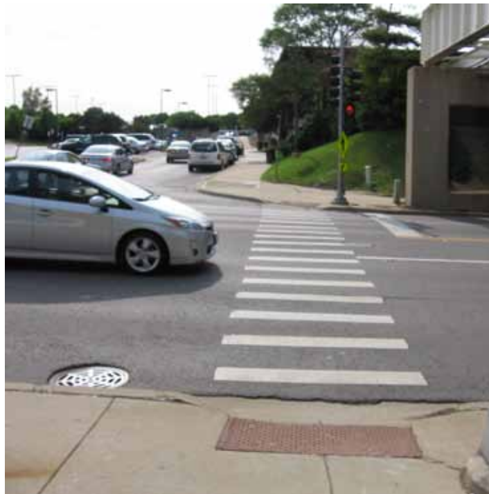
The intersection near the Des Plaines Avenue Bridge has ladder-style crosswalks and curb cuts (red) to help increase visibility of pedestrians crossing at an intersection.
