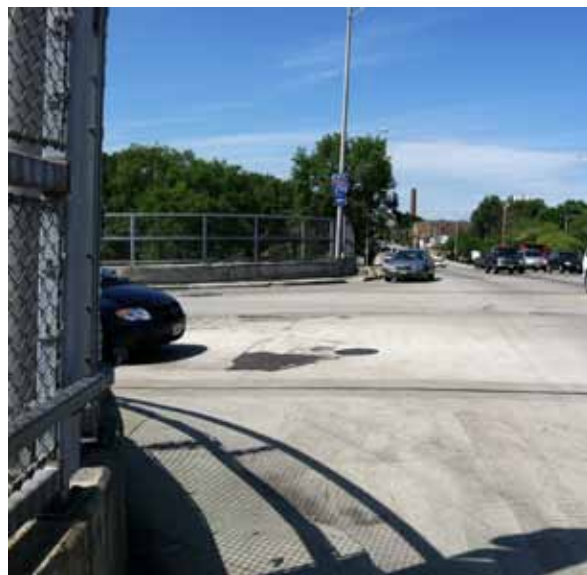
The narrow sidewalk on Harlem creates a hazard for pedestrians entering and exiting the Blue Line station.
