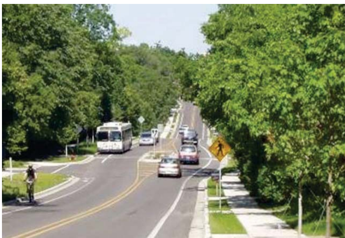
This is pedestrian flare-out style median. Diverting the vehicular traffic around the center median adds to the traffic calming effects
