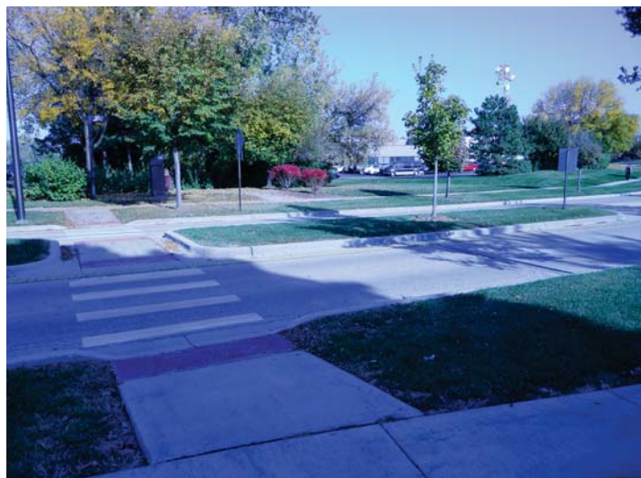
A pedestrian refuge in a median allows for pedestrians to cross one travel direction at a time.
