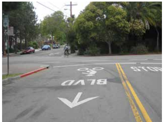
BIKE BOULEVARD PAVEMENT MARKINGS
