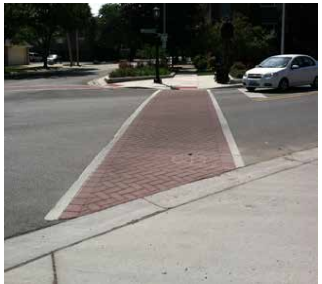
STAMPED CONCRETE CROSSWALK
