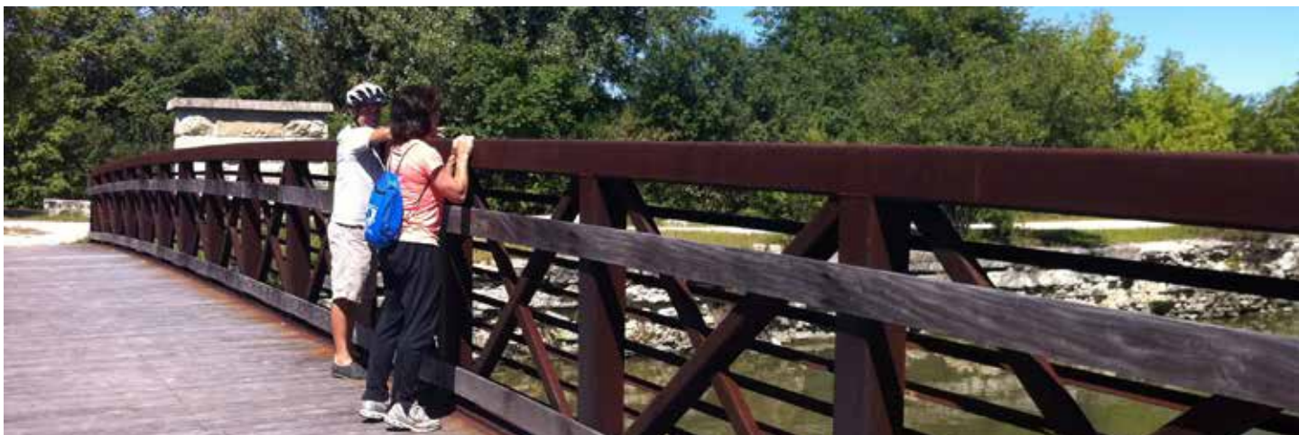
A bridge crossing over the I & M Canal in Lemont
