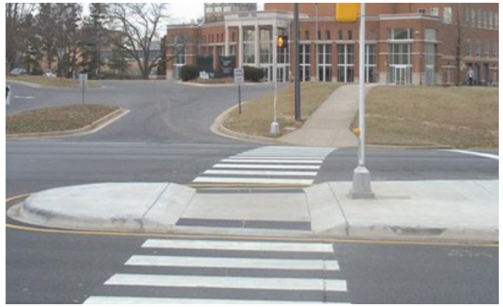
Pedestrian refuge island. Photo courtesy of North Carolina Department of Transportation.
