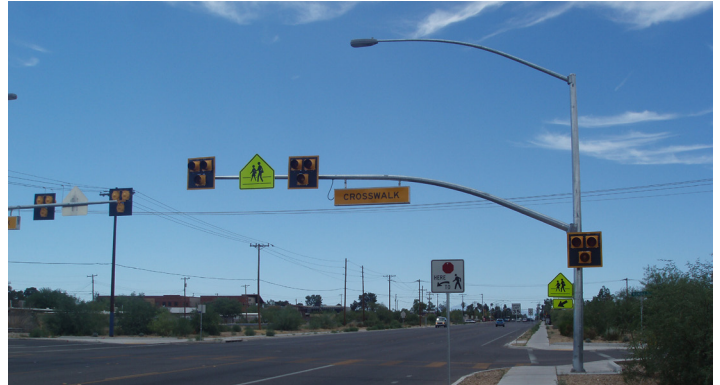
Example of a HAWK signal. Photo courtesy of the North Carolina Department of Transportation.
