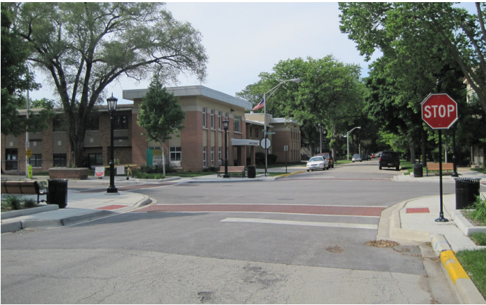
Curb extensions increase pedestrian visibility and reduce crossing distance.
