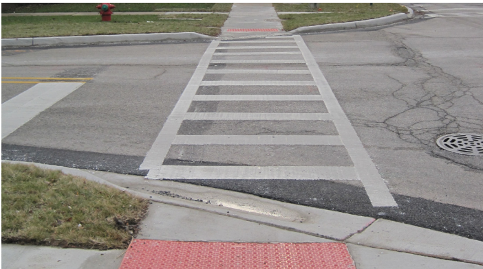
Example of a high-visibility crosswalk.
