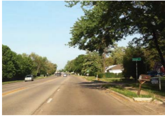
GENEVA ROAD carries heavy traffic and is a good candidate for installing side paths.
