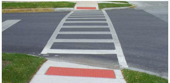
Ladder style crosswalk
