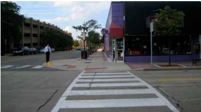
Ladder style crosswalks and bump outs make it safer for pedestrians to cross the street.
