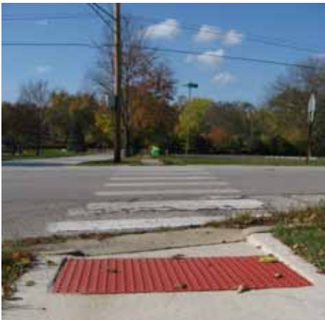
Curb cuts that meet ADA standards help people cross the street by building a ramp from the street to the sidewalk.
