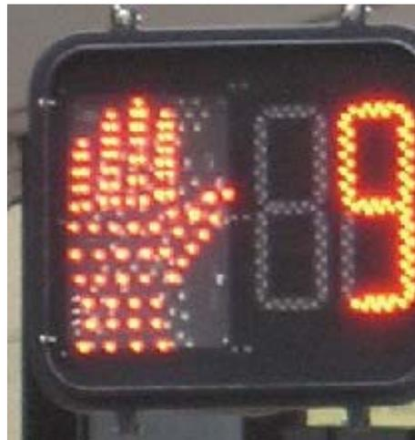
Pedestrian signals with timers convey the actual time someone has to safely make it through the intersection.
