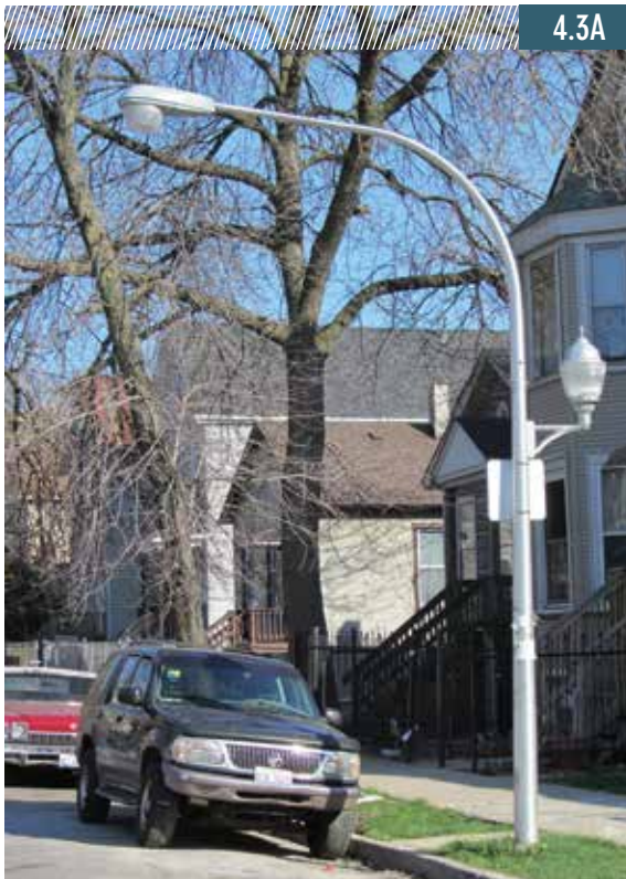
FIGURE 4.3A COMBINATION PEDESTRIAN AND STREET SCALE LIGHTING Chicago, IL
