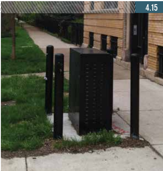
FIGURE 4.15 UTILITIES Chicago, IL
