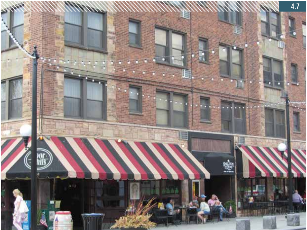
FIGURE 4.7 CATENARY LIGHTING Oak Park, IL
