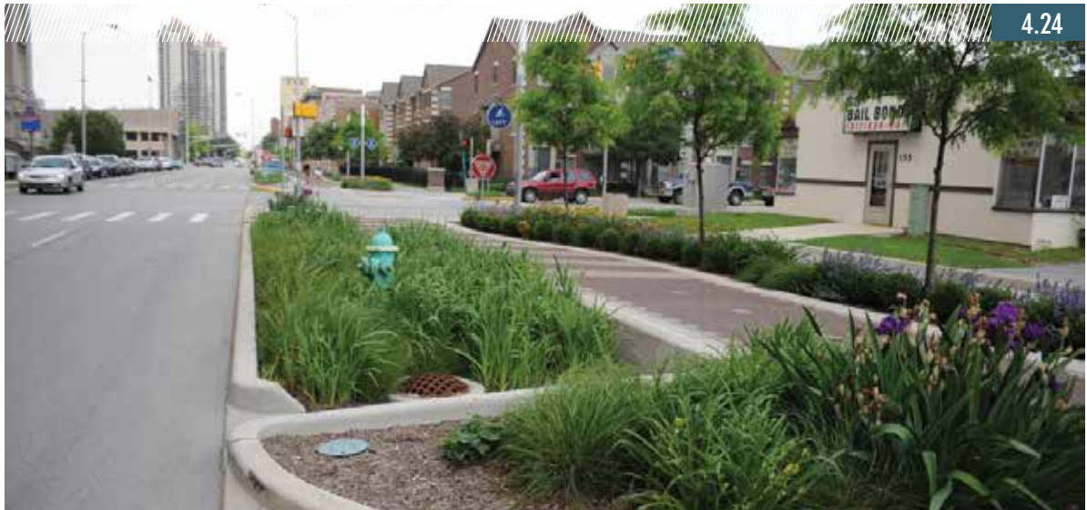
FIGURE 4.24 RAIN GARDENS Cultural Trail Indianapolis, IN Credit: Casey Jo Ailes
