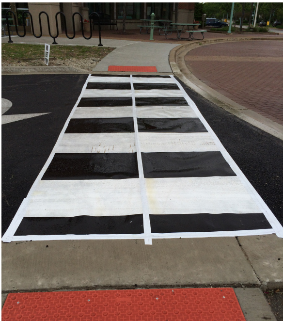
Example of a temporary crosswalk installed in Willow Springs, IL.
