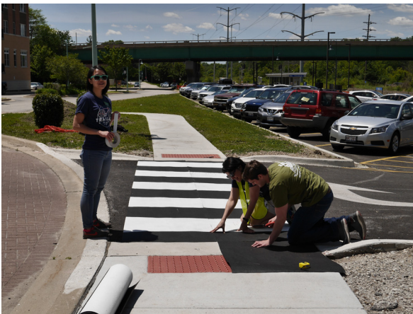
Example of a temporary crosswalk installed in Willow Springs, IL.
