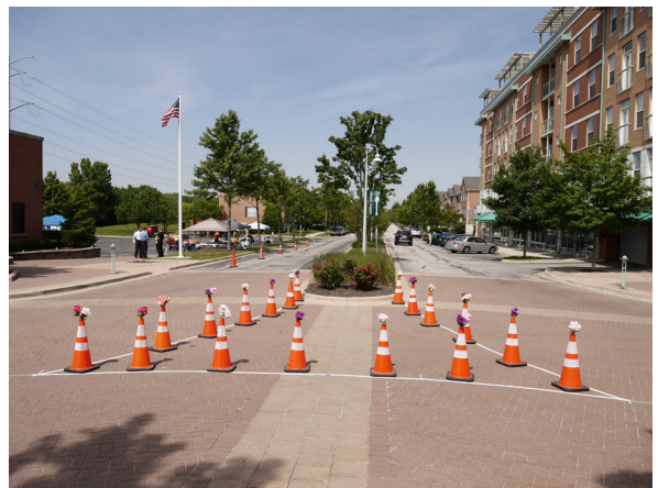
Example of a temporary bump-out in Willow Springs, IL.
